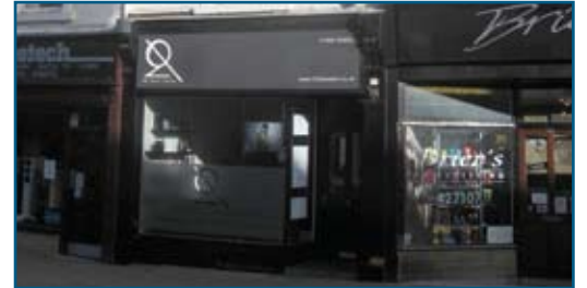
16 Cross Church Street, Huddersfield
